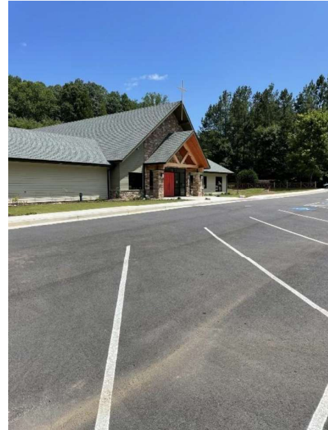
Church abutting south property line
